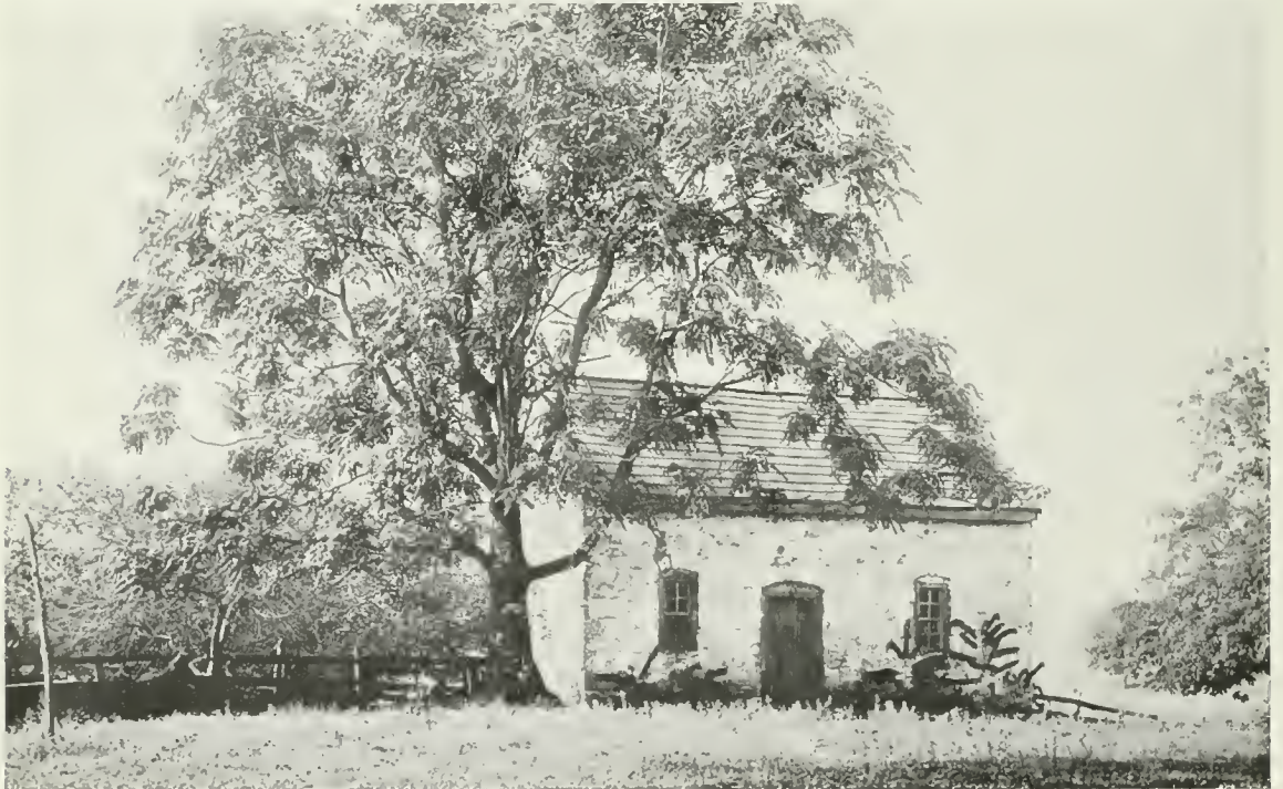
WASHINGTON'S OFFICE AT GREENWAY COURT.
